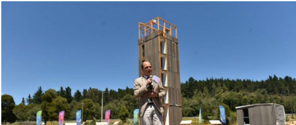
The Peñuelas Experimental Tower was inaugurated by Chile's government last year (Credit: Chilean Ministry for Housing)
