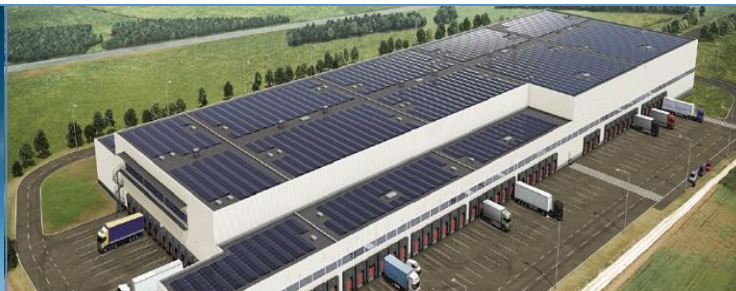
GE Hybridkraftwerk Power Conversion Berlin Marienfelde Tomorrow is made in Europe
